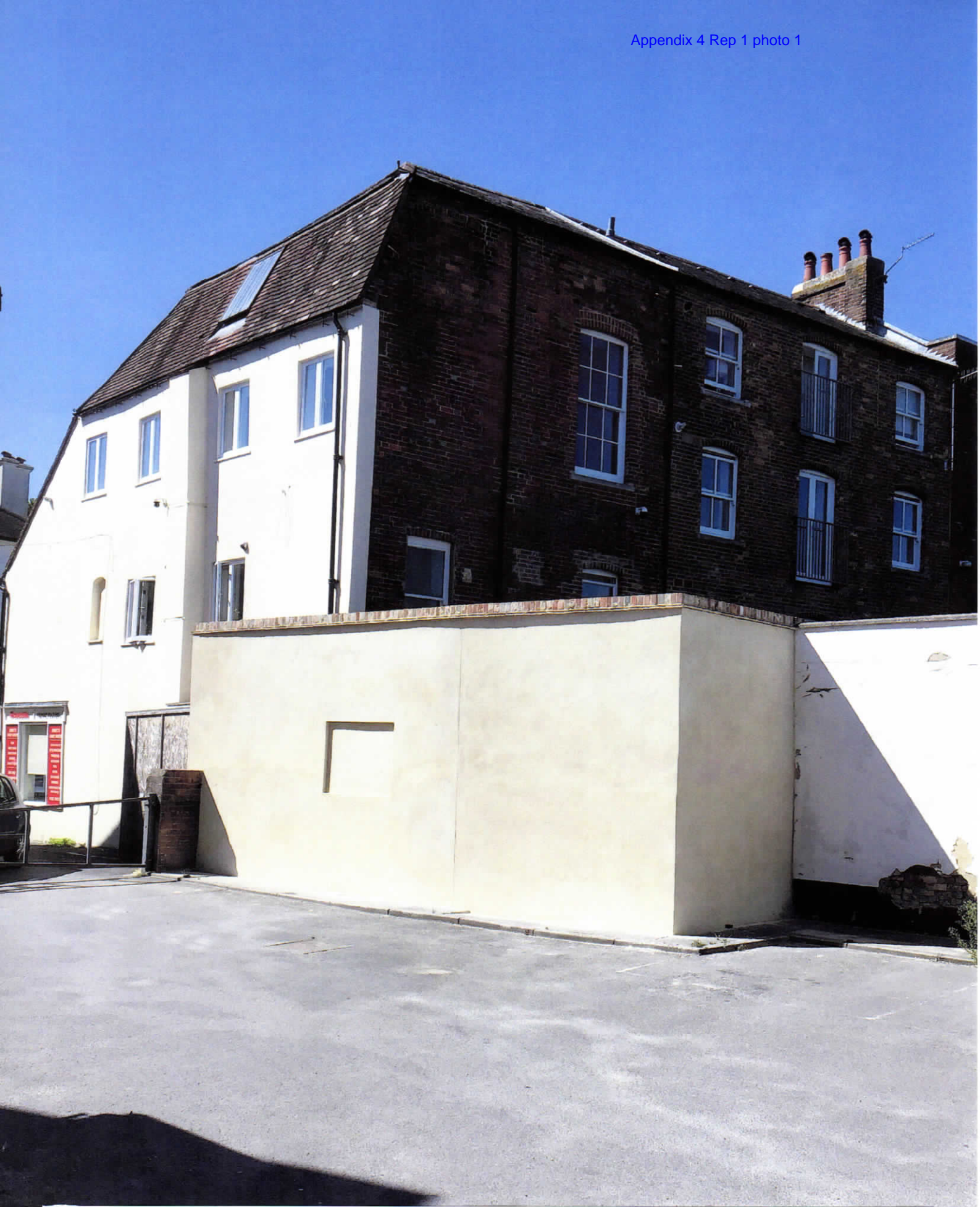
View from proposed beer garden looking towards the flats 6a, 6b, 8, 8a & 8b West Borough
